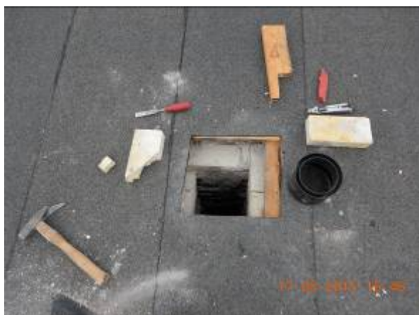
Installation of a new pipe chimney stack on Tolv-mands-barakken.
