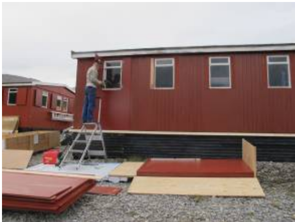
On the outside, Tolv-mands-barakken was boarded with plywood boards, which had been painted in Denmark. Afterwards the basement was strengthened with boards of the same type. New shutters were installed. These were also prepared for mounting.
