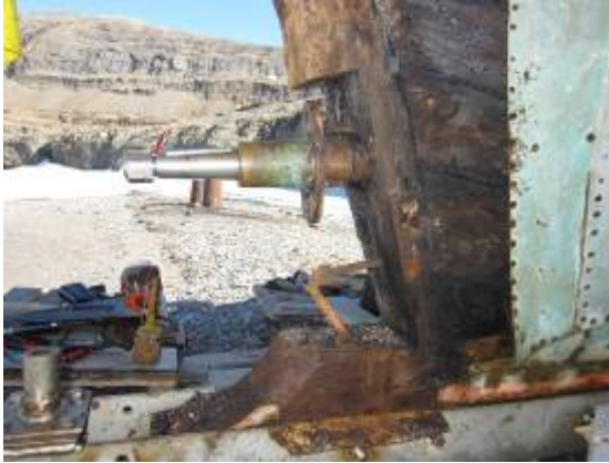
Bad wood has been chopped away
