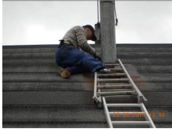
Left: The old chimney pipes in Ørnereden were completely decayed and it was only a matter of time before a conflagration could have occurred. Right: Kristian removes the old chimney.
