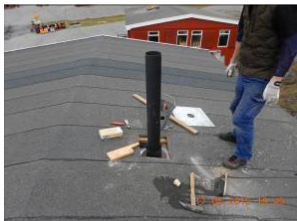
Installation of a new pipe chimney stack on Tolv-mands-barakken.
