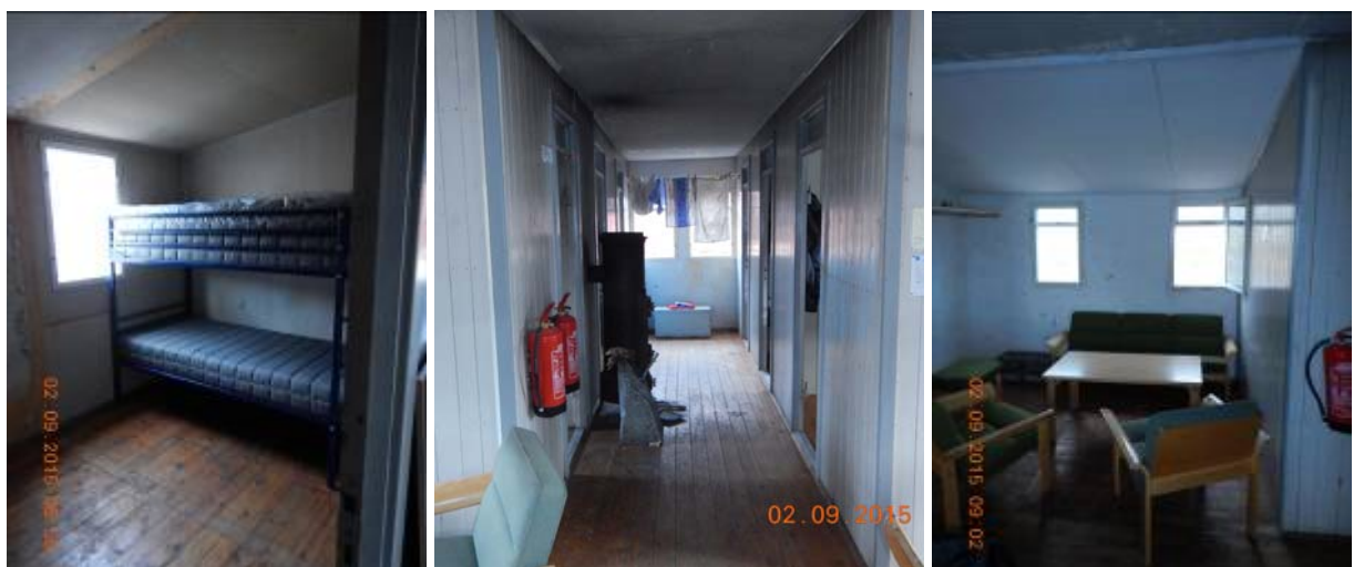
After cleaning and washing the walls and ceiling, new bunk beds were installed in Tolv-mands-barakken. In addition to kitchen /common room, the house now has 5 rooms with plenty of space for 10 people.
