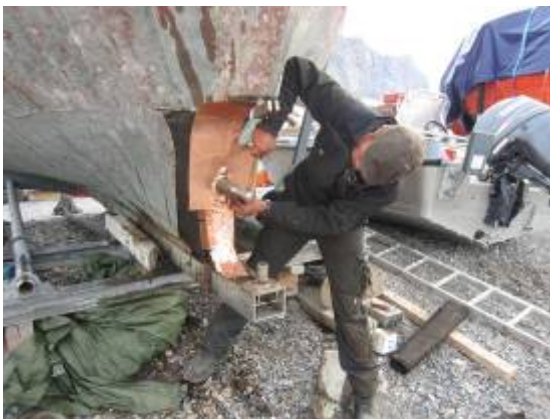
Finally new ice sheathing is attached
