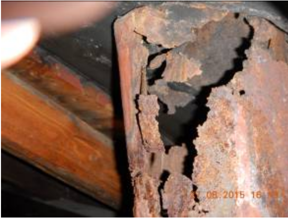
Left: The old chimney pipes in Ørnereden were completely decayed and it was only a matter of time before a conflagration could have occurred. Right: Kristian removes the old chimney.
