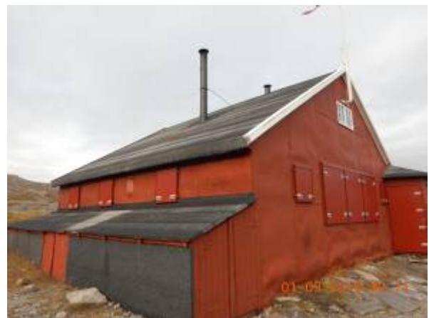
Left: Ørnereden upon arrival. Right: Ørnereden before departure. Notice the new shutters, outer door and chimney pipes.
