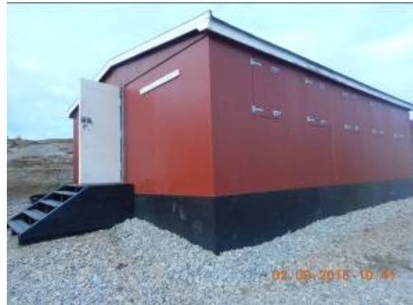
On the outside, Tolv-mands-barakken was boarded with plywood boards, which had been painted in Denmark. Afterwards the basement was strengthened with boards of the same type. New shutters were installed. These were also prepared for mounting.
